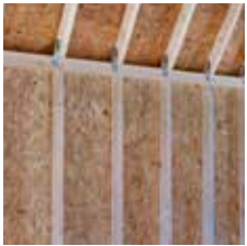
16" on-center Walls, Roof, & Floor Joists
