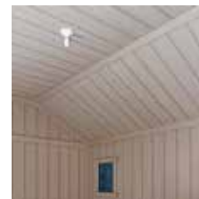
Paneling on Walls and Ceiling
